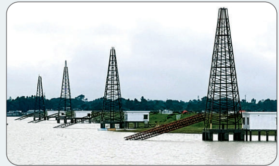
Sirajganj 2 MW Wind Power Plant under construction
