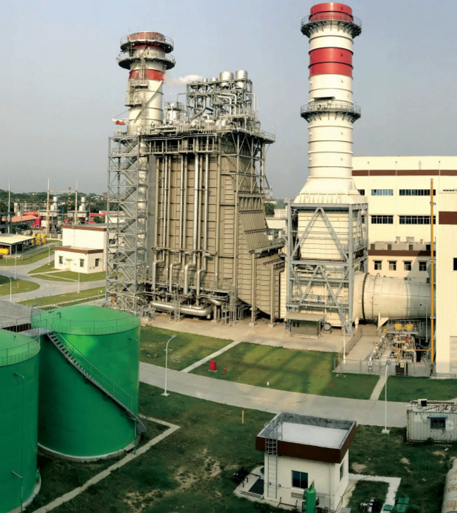
Ghorashal 365 MW Combined Cycle Power Plant
