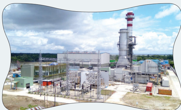
Kushiara, Fenchuganj 163 MW Power Plant
