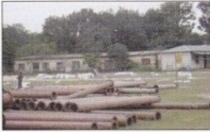
Ashuganj (Aggreko) 80 MW Quick Rental Power Plant. Expected Commissioning Date : April, 2011
