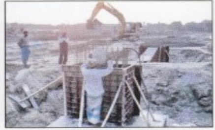
Faridpur 50 MW Peaking Power Plant. Expected Commissioning Date : August, 2011
