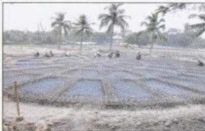
Katakhali (NPSL) 50 MW Quick Rental Power Plant Expected Commissioning Date : April, 2011
