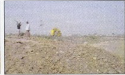
Shantabar 50 MW Peaking Power Plant. Expected Commissioning Date : February, 2012
