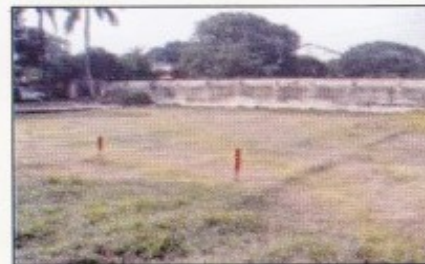
Katakhal 50 MW Peaking Power Plant. Expected Commissioning Date : February, 2012
